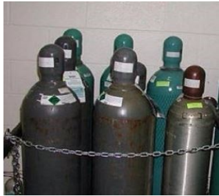
Example of proper cylinder storage
