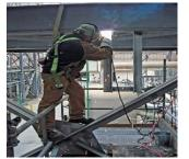
Consider alternative tie-off method (i.e. retractable to limit fall distance)
