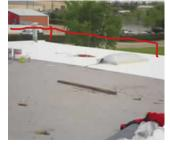
Need warning lines installed in area marked in red
